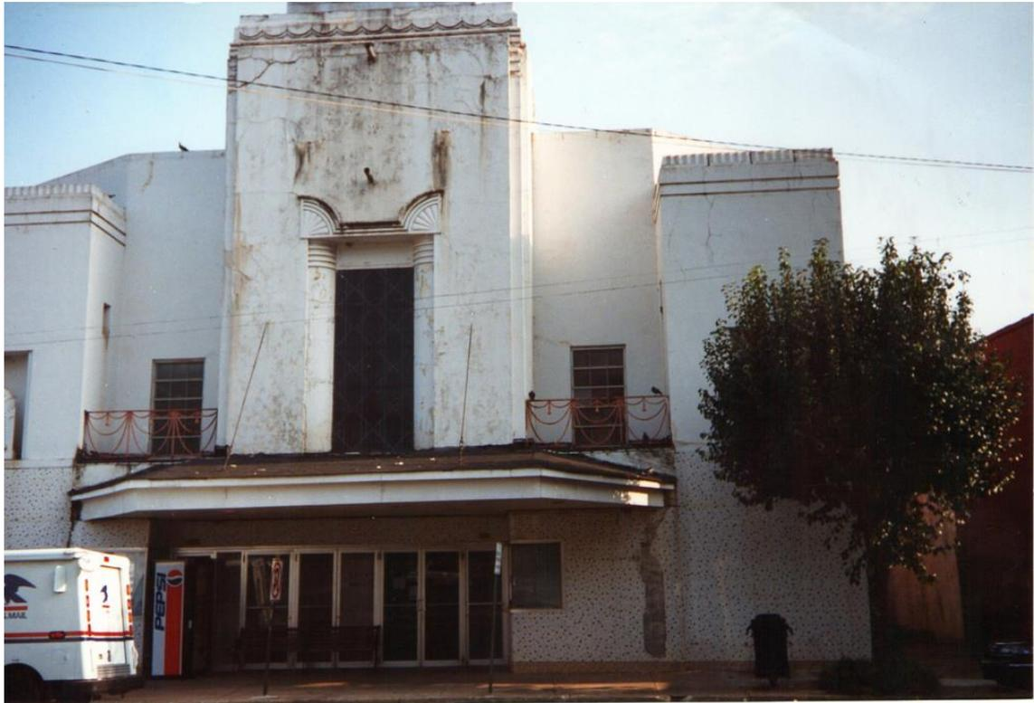
Undated photo showing much deterioration prior to the work performed in 2001-2003. Note the tile wainscot at the bottom of the façade.
