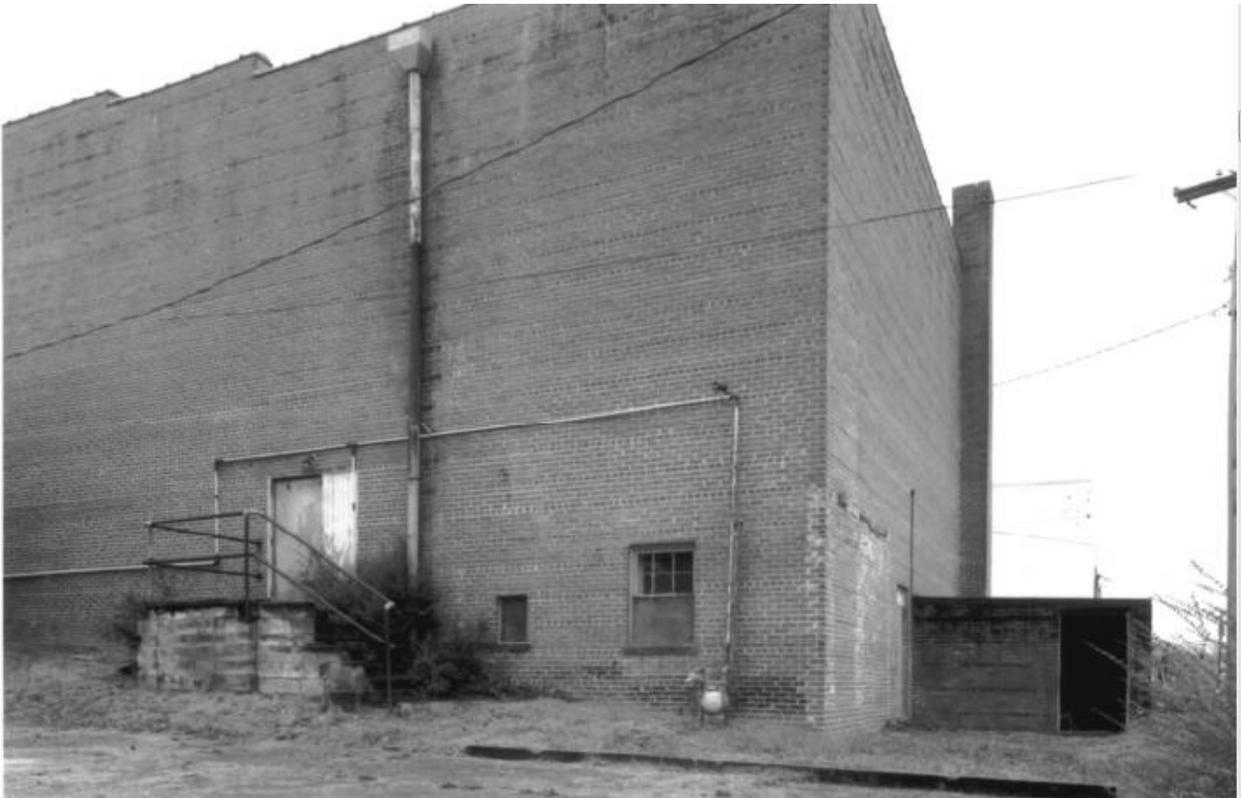
The photo of the rear of the building shows that the structure, which originally housed the cooling has been removed (far right), and that the low structure that remains housed the boilers. Other modifications include the removal of the exterior pair of doors at the top of the landing, which were replaced with a single door and infilled with wood.
