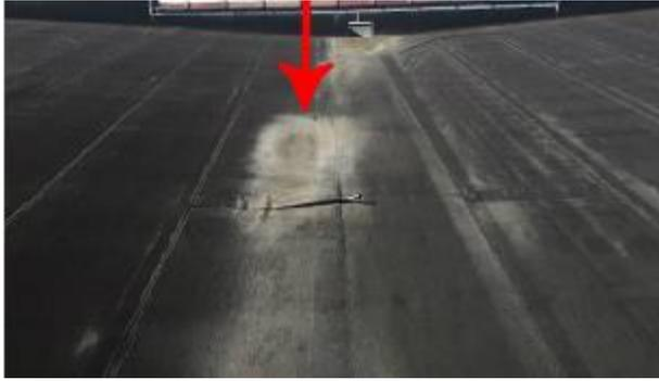
Photos at left shows the basically flat valley and stains indicate that the water ponds in the valley in lieu of being adequately directed to the scuppers.
