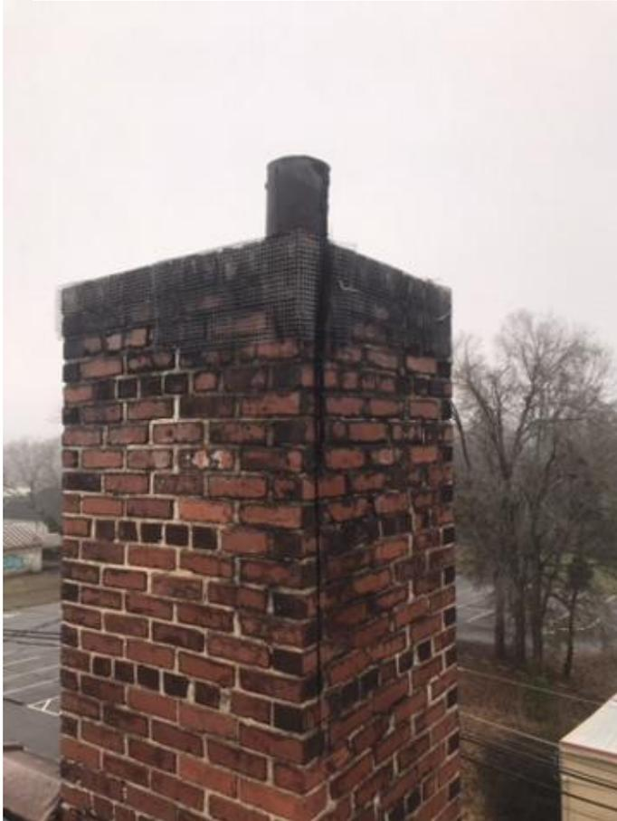
Boiler flue at left with wire to prevent rodents/birds from entering. Below is the collector box for one of the two roof gutters. The flue, which is no longer in use, enables water infiltration into the building. The collector boxes, which are not original, are inadequately sized and have rusted.
