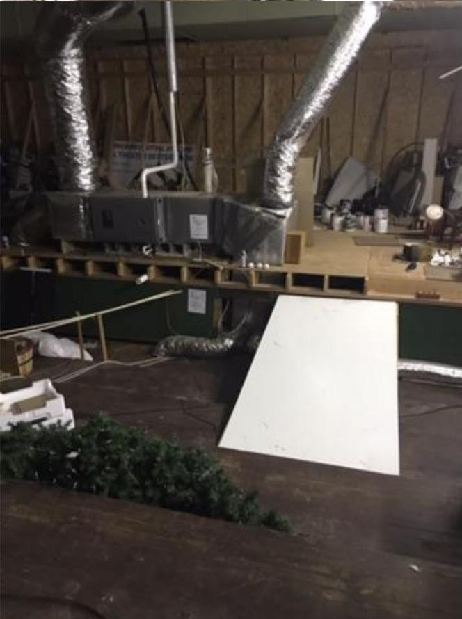
Balcony photo at left looking out over the added City Hall ceiling. The HVAC units are not in a rated room.
