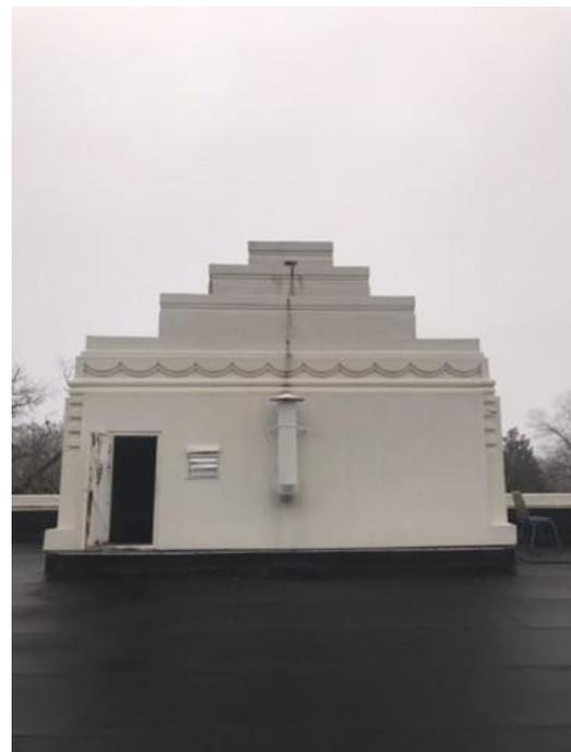
Exterior photos showing the restored masonry stucco which has held up well although there are some cracks that need addressing. Note the original tile wainscot is gone.
