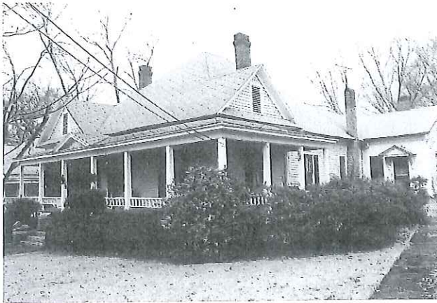
This house exhibits four properly-maintained brick chimneys that contribute to the building's architectural character.
