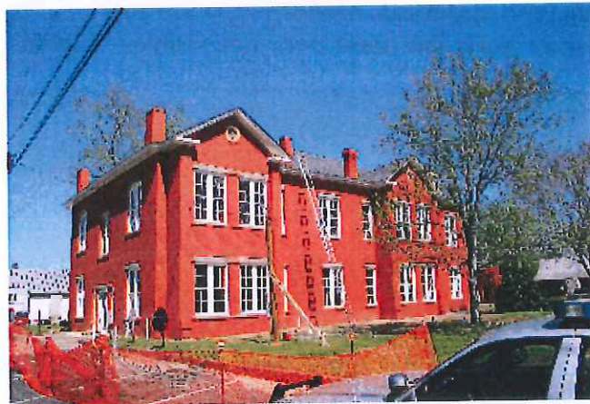
Historic Courthouse and Grounds Restoration
